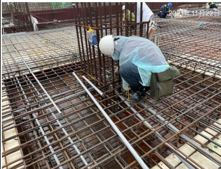
A construction worker in a white hard hat and safety harness is working on a large, horizontal steel rebar cage for a slab. The cage is made of many horizontal and vertical bars. The worker is crouching on the right side, facing the cage. A timestamp in the top right corner of the image reads "2021年11月22日".                                                                                       | <p>拍攝日期：<br/>110 年 11 月 22 日</p> <p>地點：<br/>A4 區 1F 板</p> <p>說明：<br/>1F 板 RC 消防配管</p>   |
